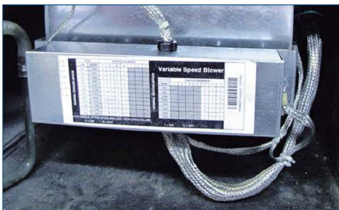
Figure 6 — After I knew that shielding the wiring harnesses would suppress the EMI, I applied braid tubing over the wires to produce a more professional looking result. Note the shield grounding strap on the right side of the unit.
